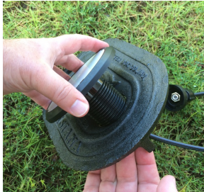
Figure 5 – Insert the Antenna into the Pit Lid
