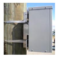
Figure 68 – UPS Attached with Clamps
