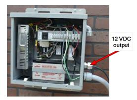
Figure 73 – 12 VDC Output Wired
