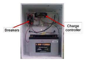
Figure 50 – Activating the Battery
