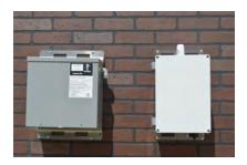
Figure 71 – UPS Mounted on a Wall
