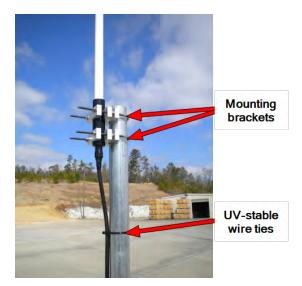
Figure 33 – Mounting Brackets
