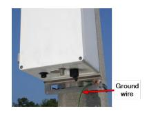
Figure 63 – Attach Ground Wire
