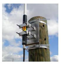
Figure 54 – Coaxial Cable Attached
