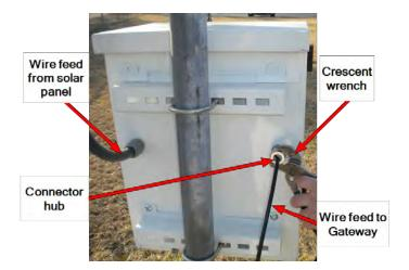
Figure 44 – Connector Hub
