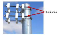
Figure 81 – Mounting Brackets
