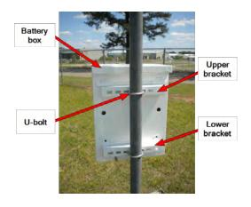
Figure 35 – Battery Box Installed
