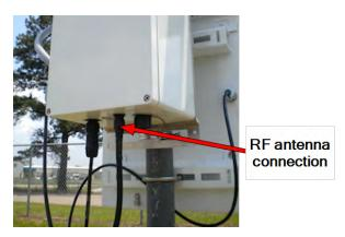
Figure 47 – RF Antenna Cable
