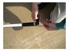
Figure 32 – Weatherizing the RF Antenna
