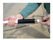
Figure 31 – Attaching the Coaxial Cable
