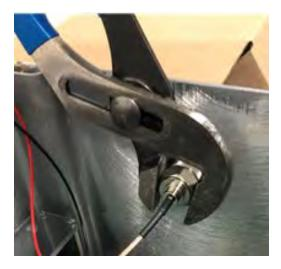
Figure 118 – Remove Existing External Cellular Antenna
