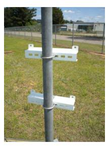
Figure 34 – Installing Pole Brackets
