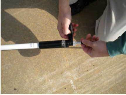
Figure 32 – Weatherizing RF Antenna
