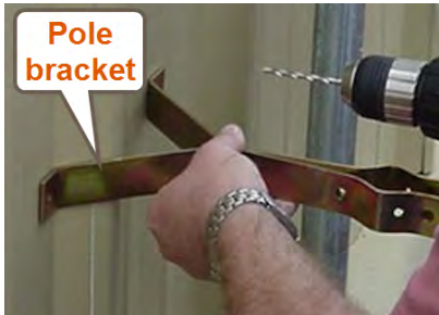
Figure 79 – Securing Pole Bracket
