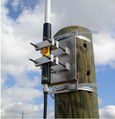
Figure 54 – Coax Cable Attached
