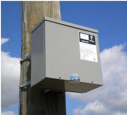
Figure 67 – UPS Attached to a Large Pole
