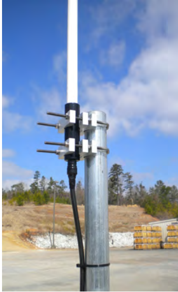
Figure 84 – RF Antenna to Mast
